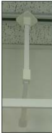
Detail of Suspending the OTRT track into an existing track. 100% Aluminum, comes in 2foot lengths, field cut to desired length
